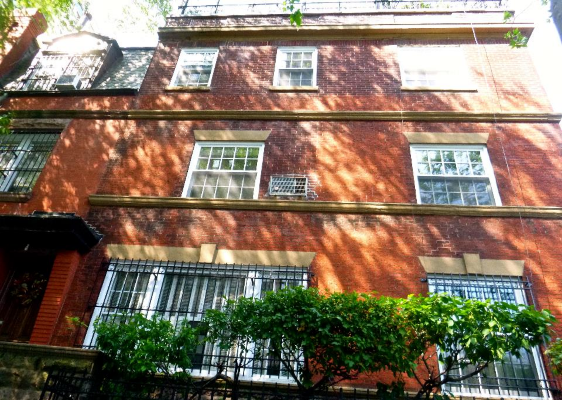
The old design of the windows of the Henderson Place. They are split up into small panes.
