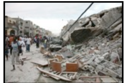
This picture was taken after the earthquake.
